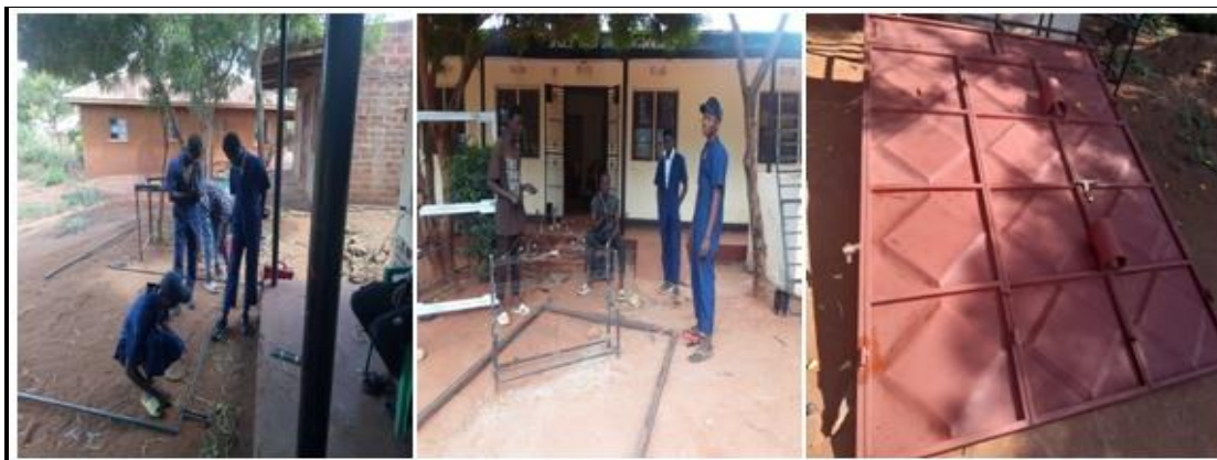
Photo 5: On left side and middle student are making door and on the right side there is a gate made by them.
